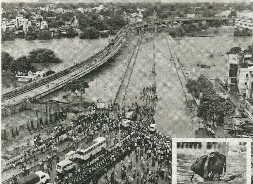
Flooding at Adyar river as seen from Maraimalai Adigal Bridge during 2015 Chennai floods; (inset) a man moves to safe place from Kotturpuram in 2015 | EXPRESS/ PTI
