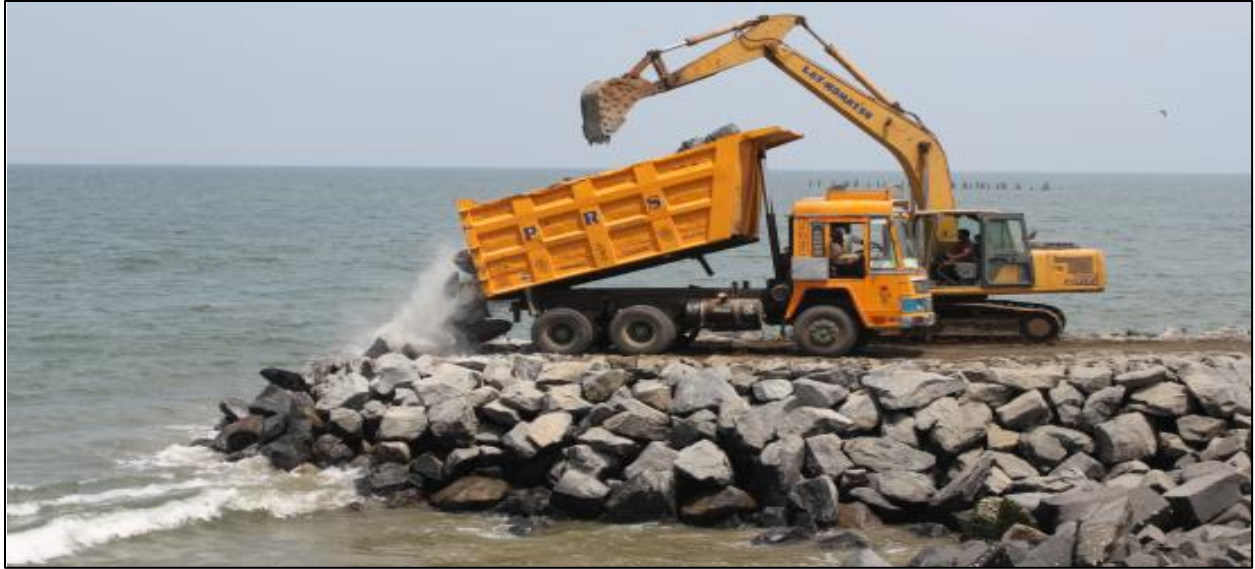
Construction of working platform and reef base
