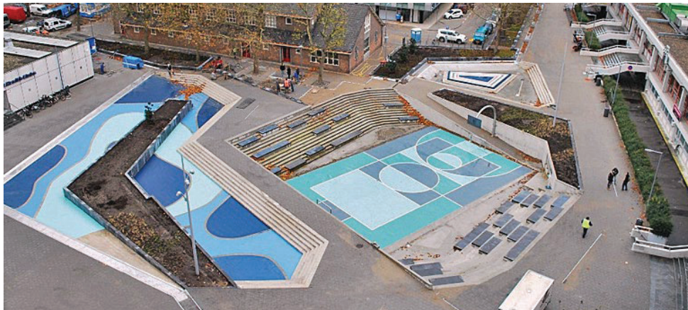
New innovative water square combines leisure and storm water storage in Rotterdam, the Netherlands
