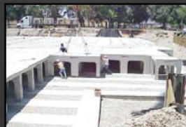
Construction of 1.7 acre infiltration chambers which are 5
