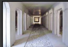
Underground infiltration chambers at
