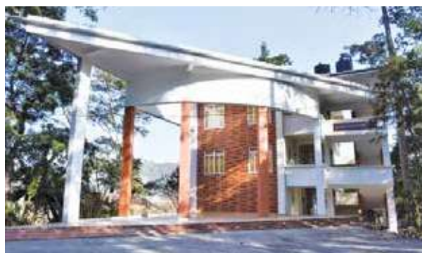
Newly Constructed Academic Building, SFTI, Aizwal, Mizoram
