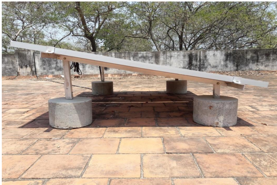
Figure 2.22: Photograph of the Solar Panel mounted in the EEE Department of PEC
