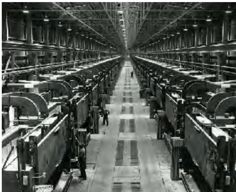
Figure 3-18: Soderberg Electrolytic Cell Line - Kaiser Chalmette Plant
