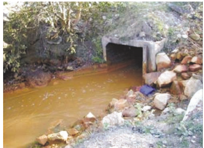
Mine Drainage Water
