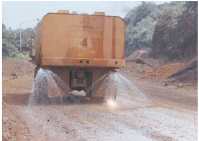
Water Sprinkling on Road for Dust Suppression
