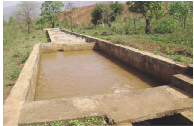
Settling Tanks to Treat Mine Water
