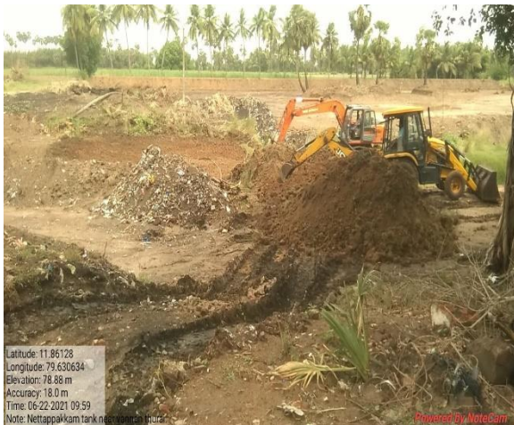
Nettappakkam tank Before
