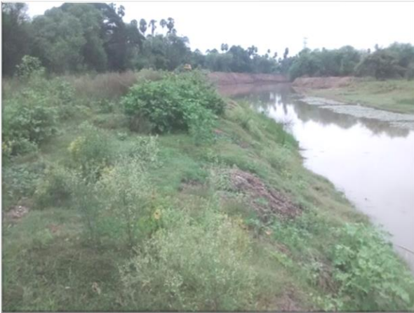
Katterikuppam tank Before
