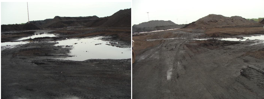
Photo Nos. 4, & 5: Status of coal storage, water stagnation and undulance of the floor
