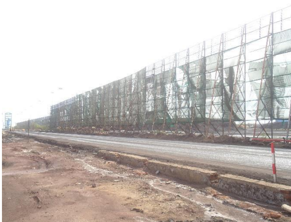
Photo No. 18: Wind Screen first barrier from Coal yard
