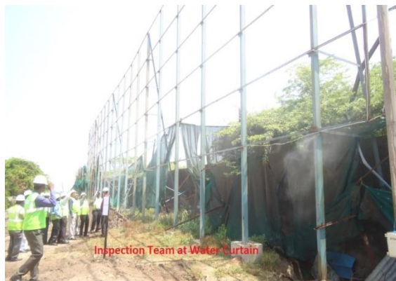
Photo-20 Water Curtains under trial run
