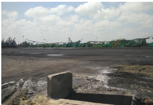
Phpto-19 Partially damaged Wind Screen towards Keezhavanjore
