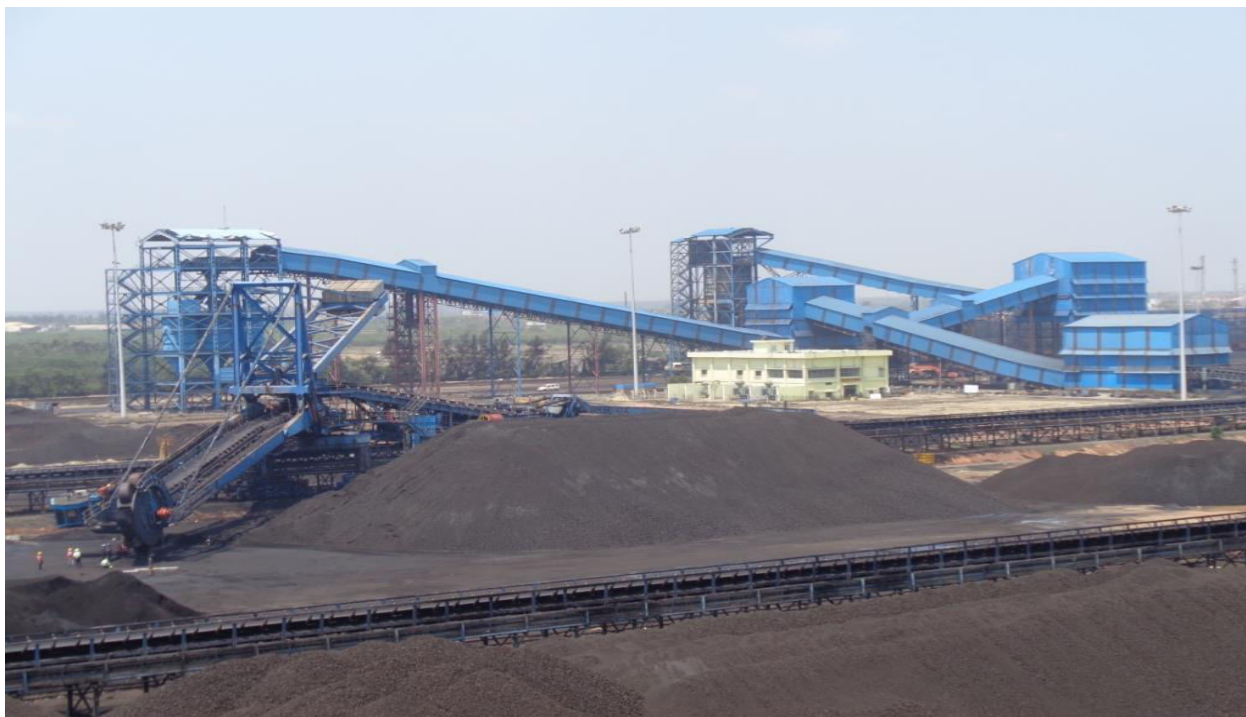
Plate-5 Overall View of Reclaimer /Stacker, Closed Conveyers, Transfer Towers and Coal dispatch to Truck & Wagon
