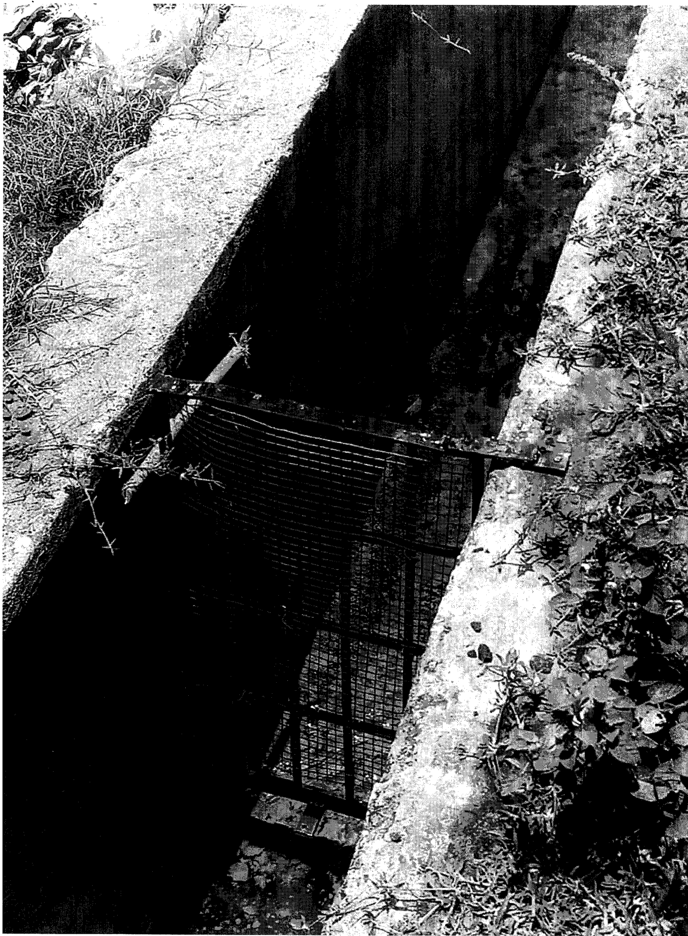
Vambamedu 'U' drain near culvert crossing
