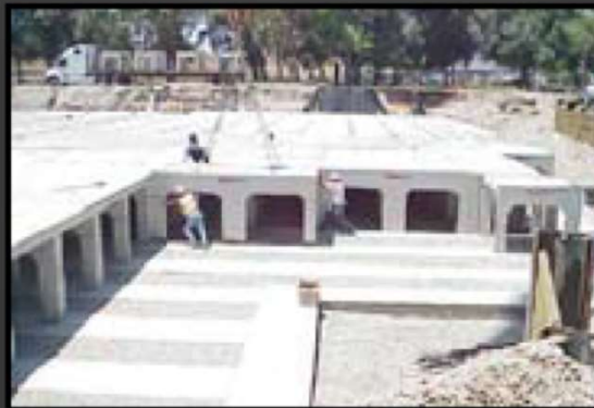
Construction of 1.7 acre infiltration chambers which are 5
