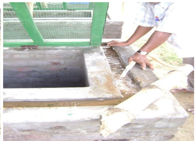
SATURATING FILLED SAND
