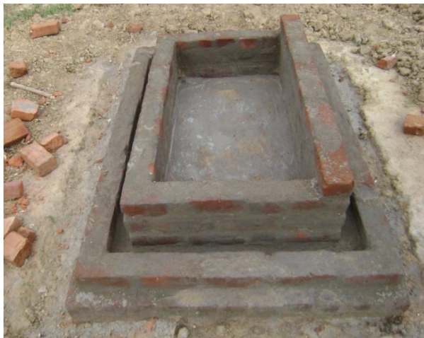
DOUBLE WALL CONSTRUCTION
