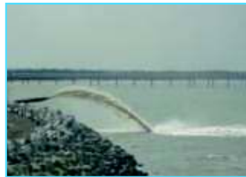
Sand bypassing – north side
