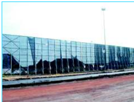
Fabric barrier along the coal stock pile
