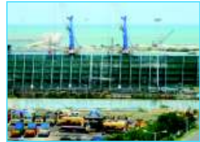
Fabric barrier erected to arrest the dust particles carried by the wind outside the port
