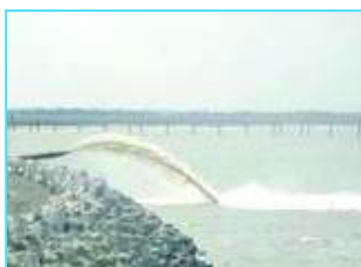
Placement of sediments for beach nourishment
