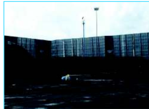
Inside view of the coal stock area surrounded by Fabric barrier
